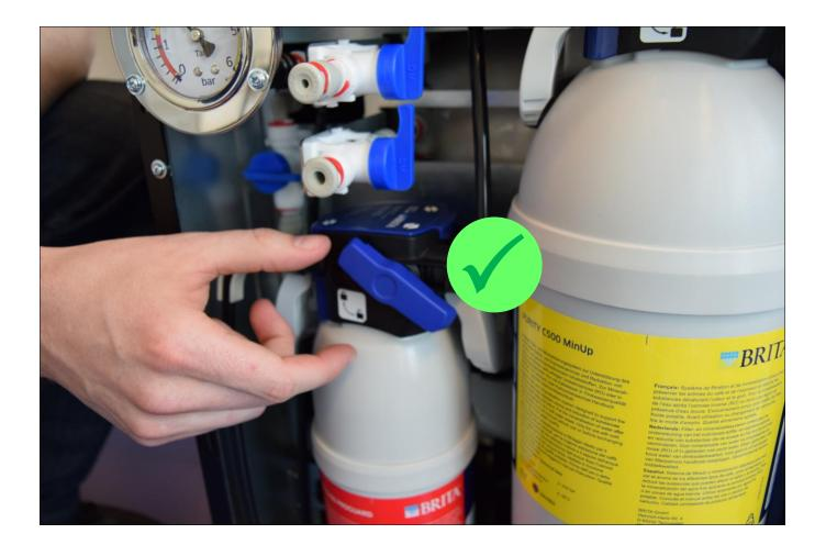
Open the sampling valve Empty the storage tank Close the sampling valve
